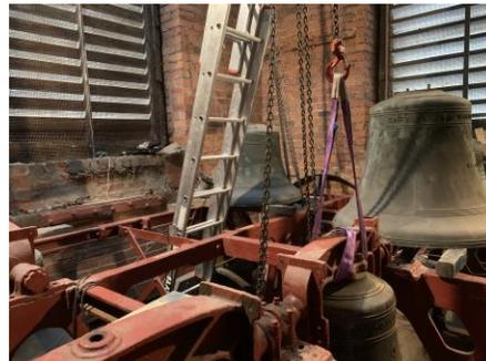
some of Penn bell ringers and the bells in various stages of removal from the frame. There are views of the bell chamber and ringing room, with block and tackle sets used for lifting and lowering the bells and heavy fittings. One shows the remains of a leather washer from a bell, greatly worn after ninety years use. Headstocks and clappers are lined up ready to go for renovation.
